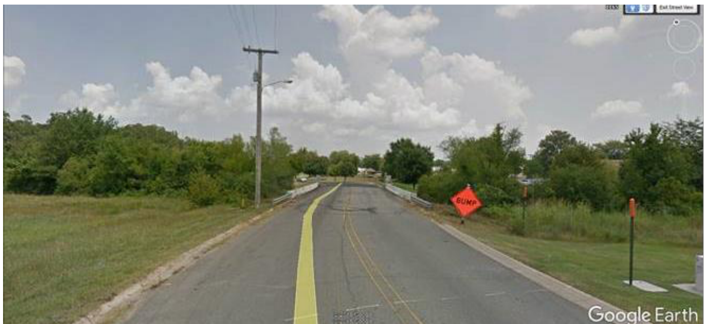
Figure 7. Bob Courtway Bridge to Be Widened
