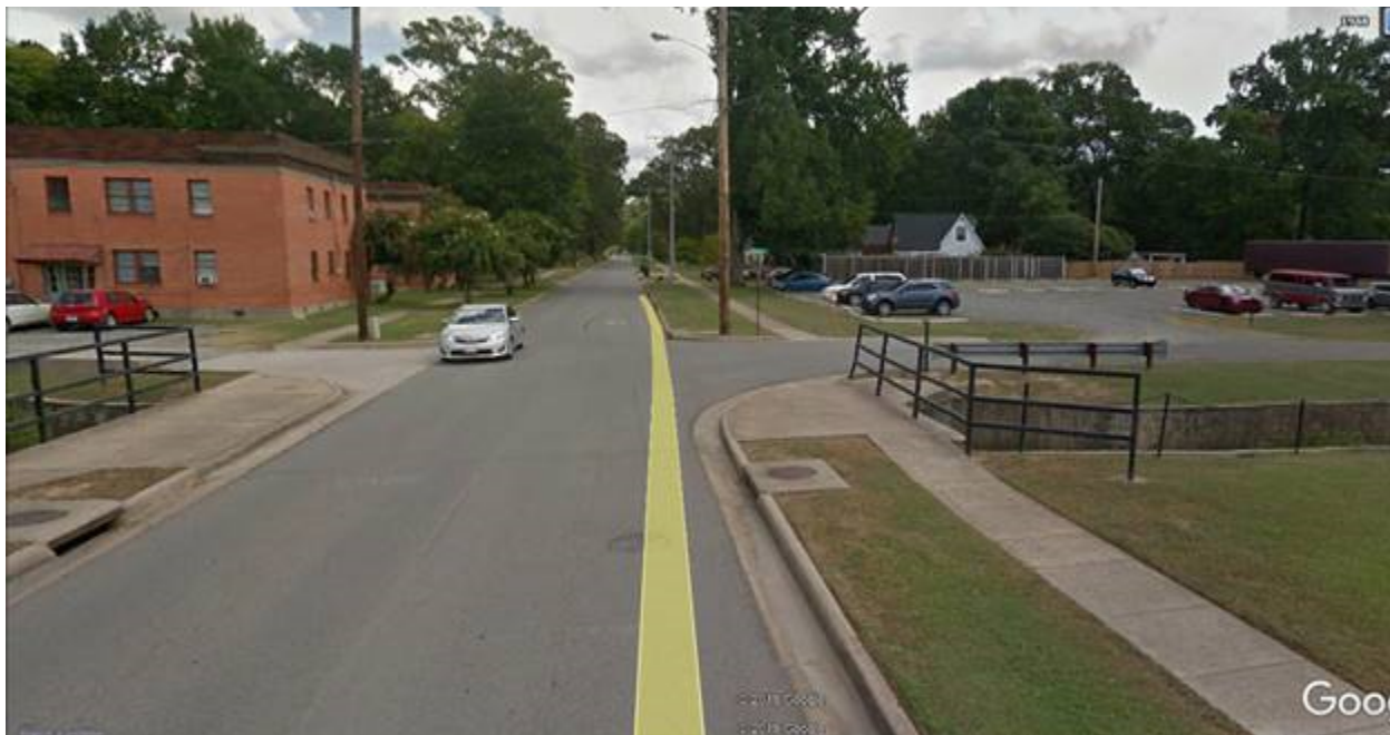
Figure 5. Site of Box Culvert to Be Installed Between Donaghey Avenue and Bruce Street
