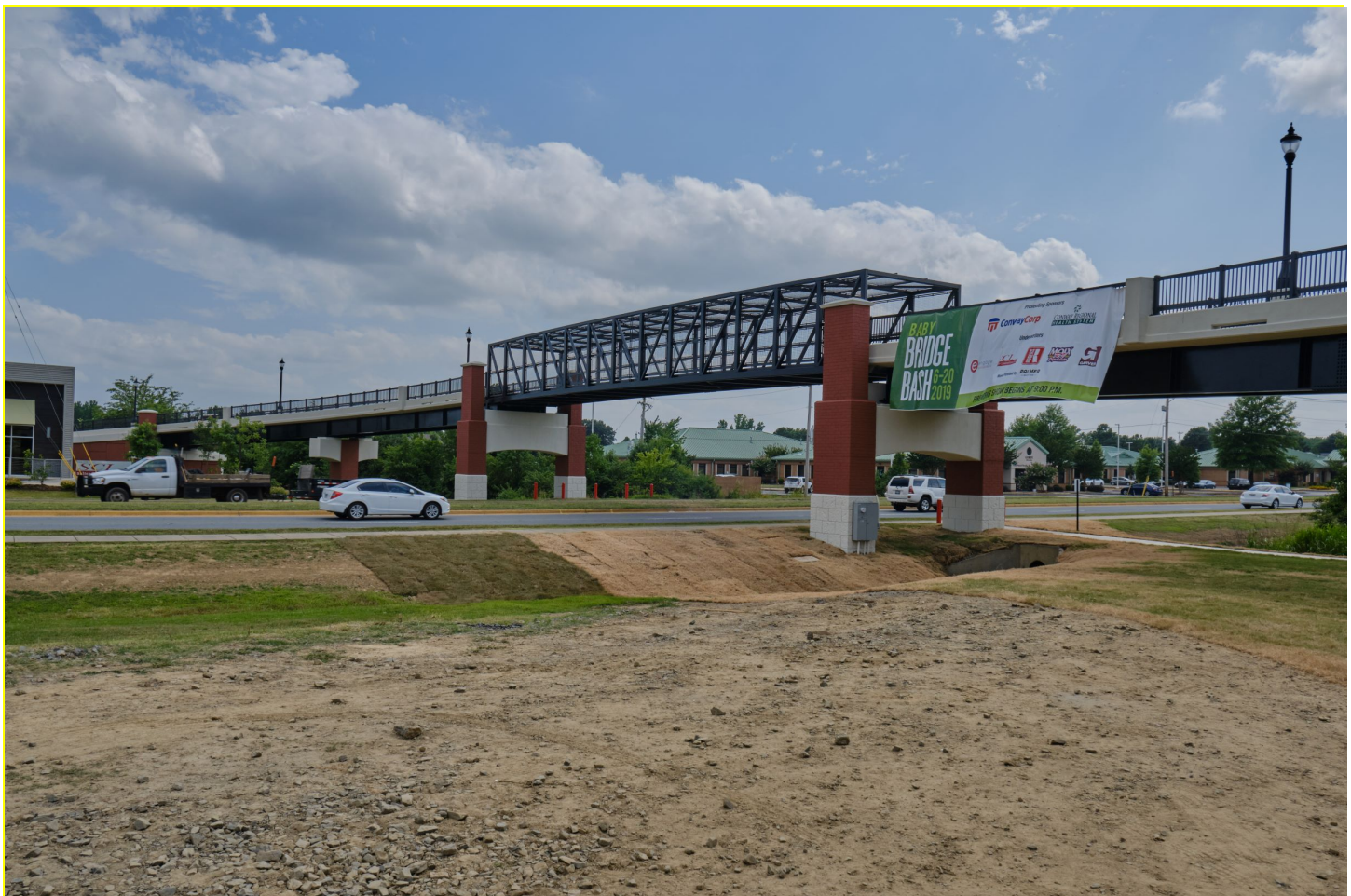
Figure 2. Newly constructed 6 th Street Bridge
