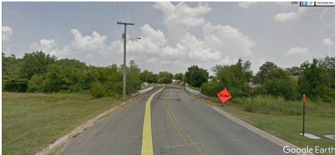
Figure 7. Bob Courtway Bridge to Be Widened
