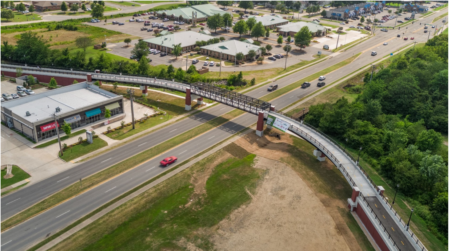
Bicycle-Pedestrian Bridge Over Dave Ward Drive
