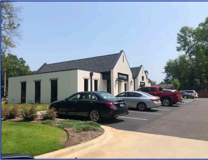
View of site from Caldwell St looking SE
