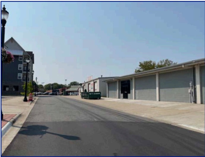
View of the site from Smith St looking W
