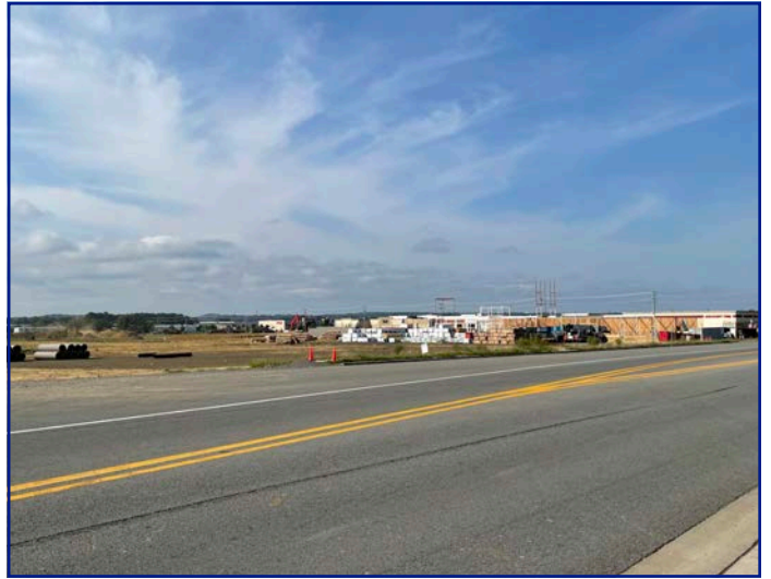
View of hotel construction from E Dave Ward Dr looking SW
