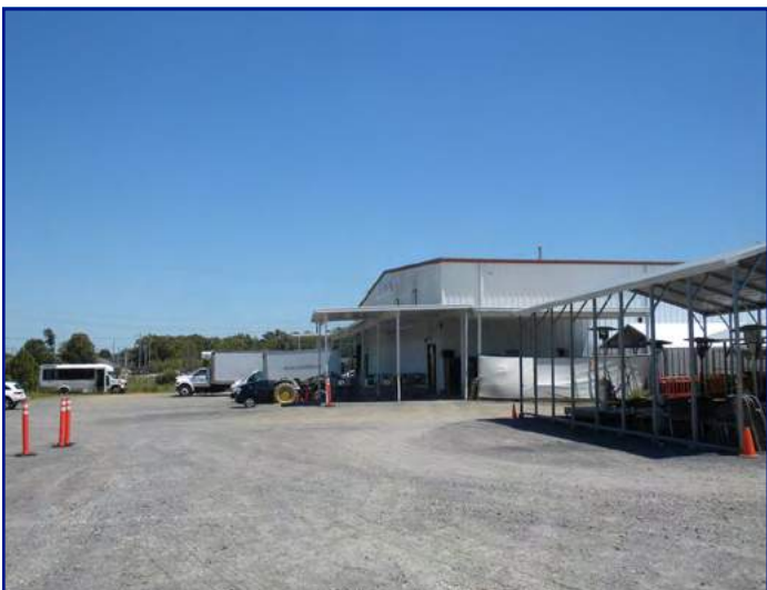
North and west façades of main building with new canopy; accessory structure
