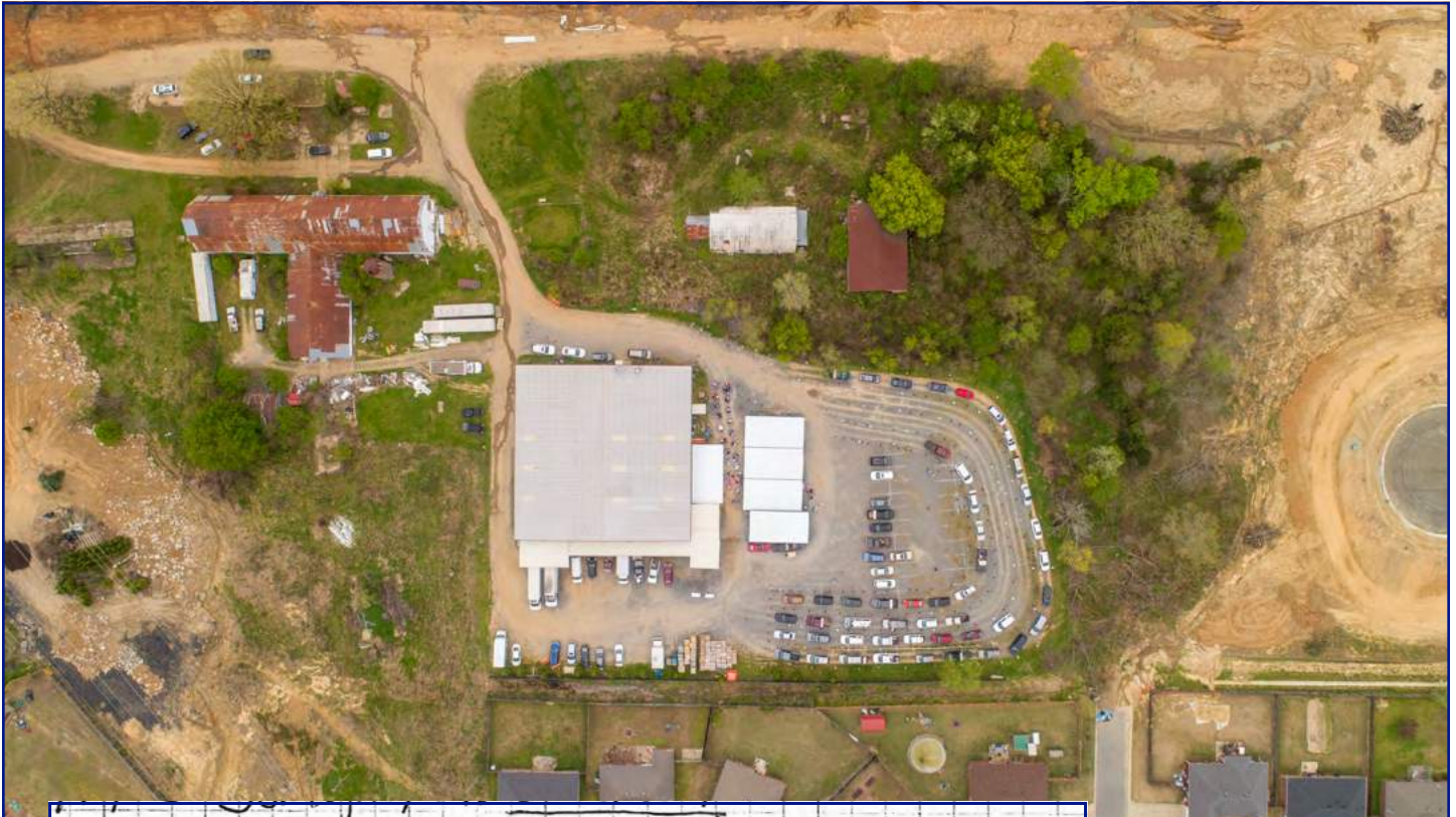
Applicant provided aerial photo of site
