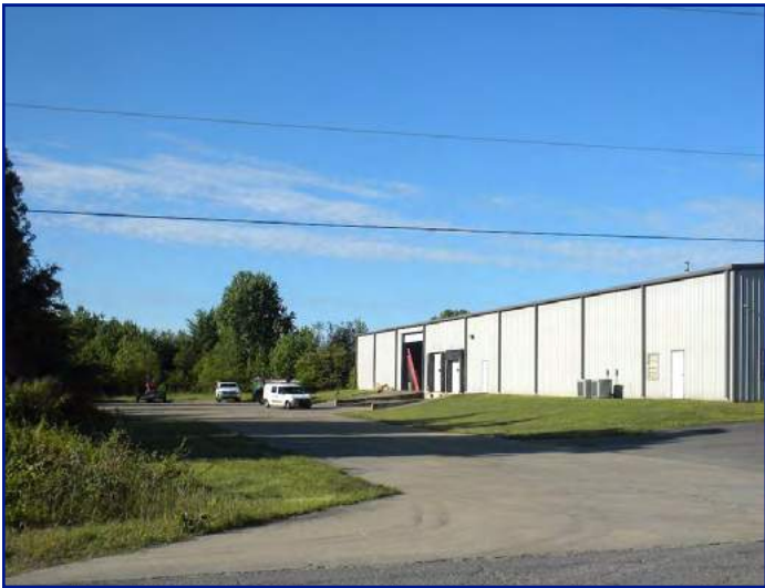
N façade of Coney Garage Doors/C&S Guttering; proposed access to mini-storage site
