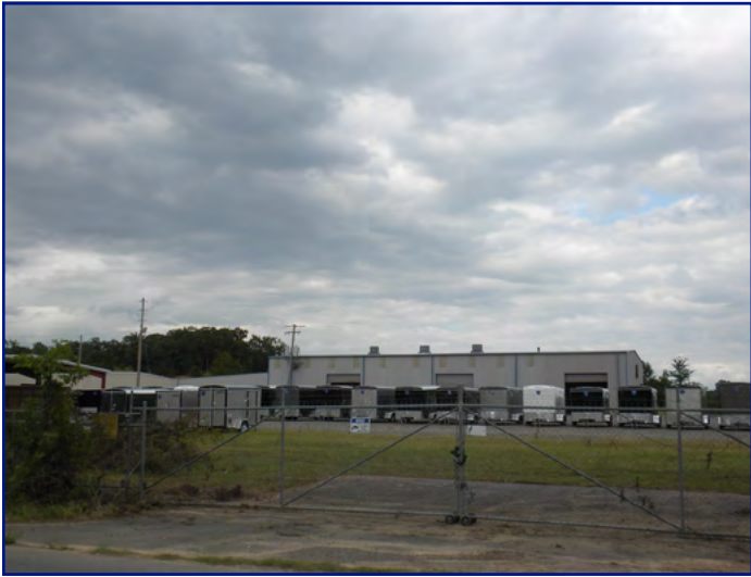
View of subject property from McNutt Rd looking E
