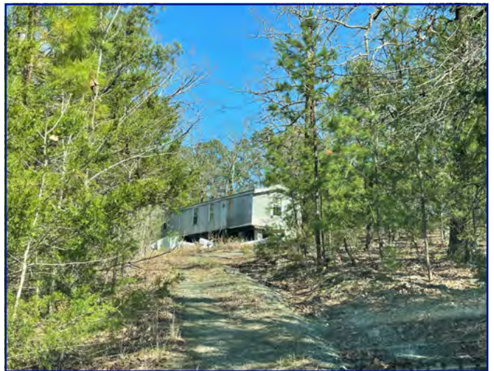
View of subject property from Ridgedale Cir looking E
