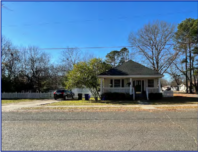
View of subject property from Mitchell St looking W
