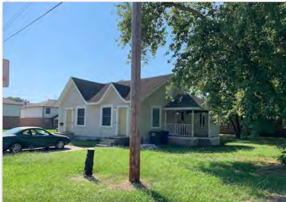
View of abutting properties across Martin St panning [L to R] SE to SW
