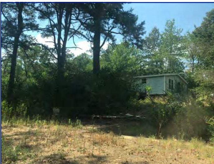
Property adjacent to the N
