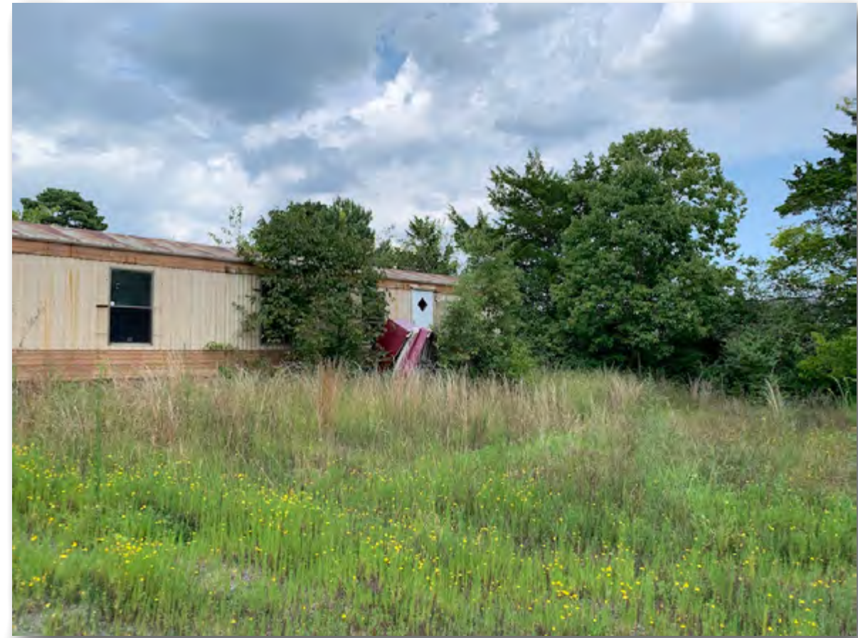
Single-family residence, to be removed
