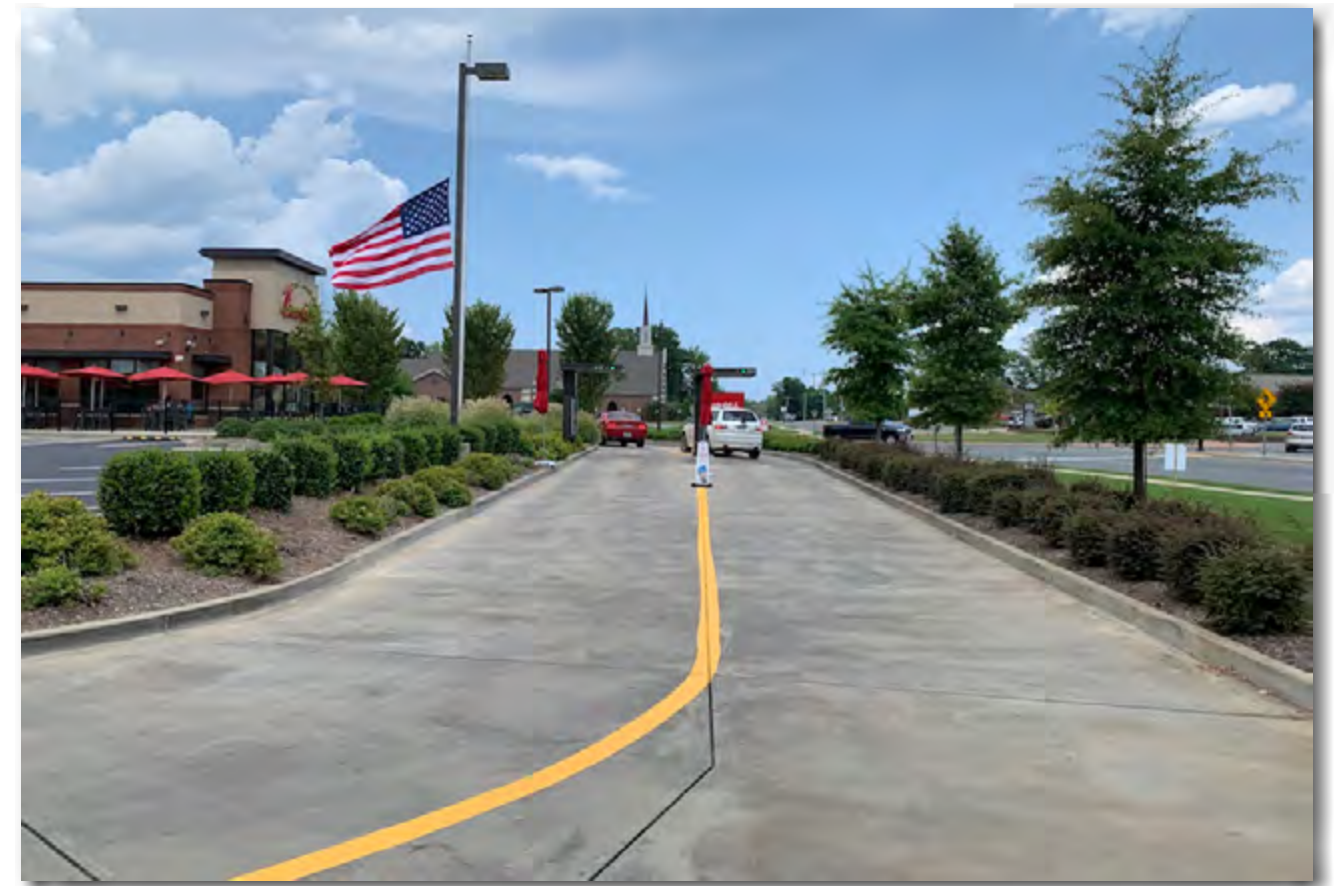
View of existing drive-through looking E
