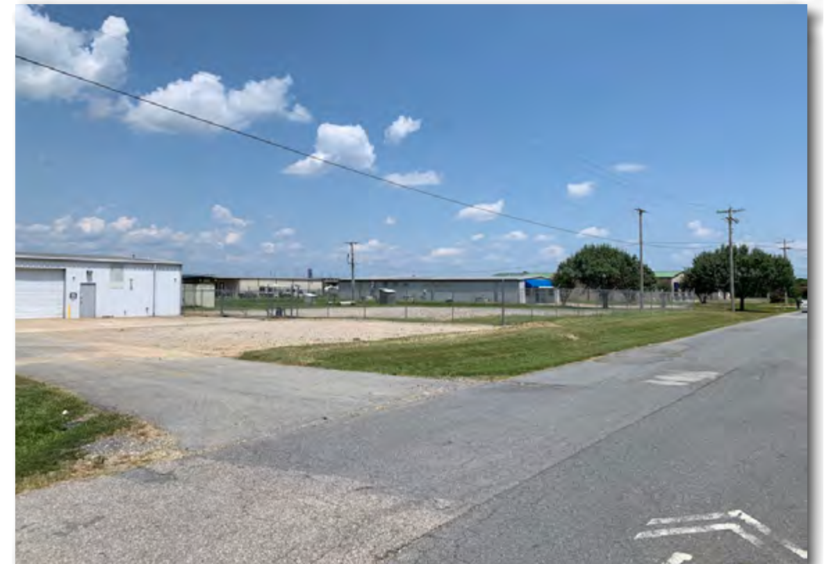
View of property from Jeanette Dr looking NE
