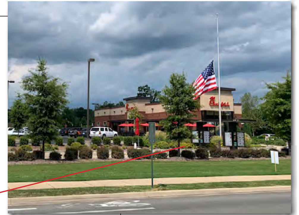
View of existing drive-through from Prince St looking NE
