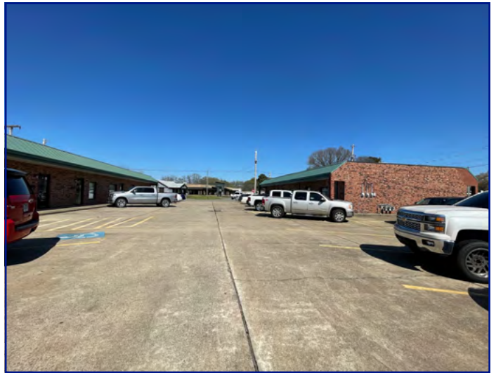
Remainder of development to the E; Court St and Harkrider St beyond
