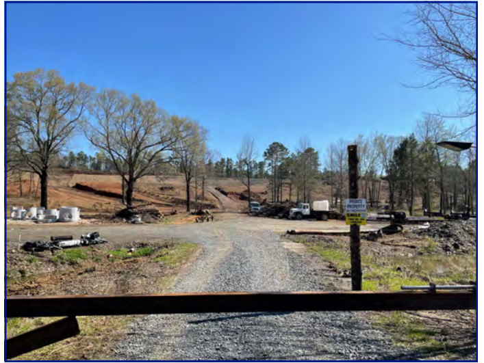
View of subject property from access road looking S
