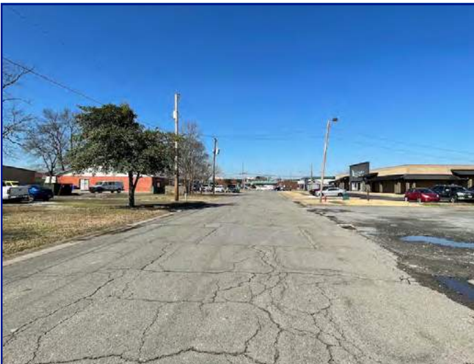
View of 2nd St looking W
