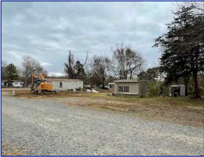
View of subject property from Azalea Ln looking SE
