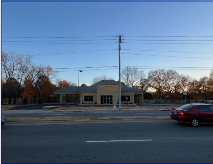
View of subject property from Prince St looking S
