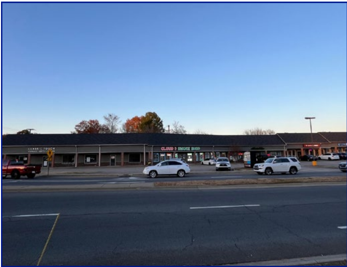
Property adjacent to the N
