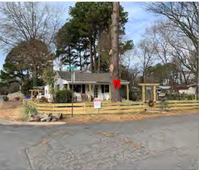
View of subject property from Western Ave looking west
