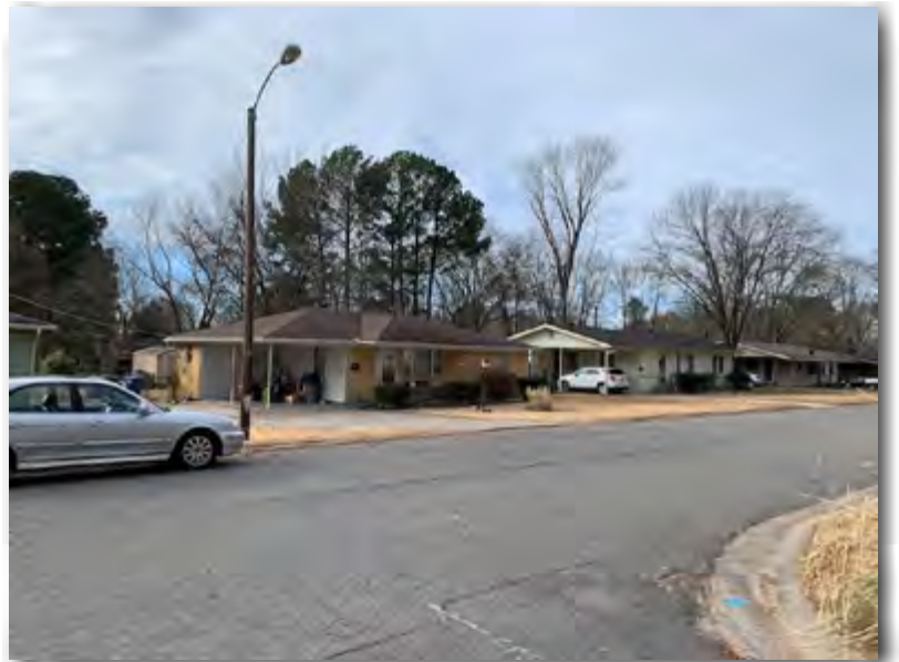
View subject property/Western Ave looking southwest
