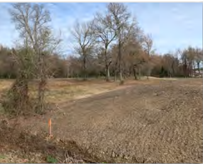
View of site work to increase elevation
