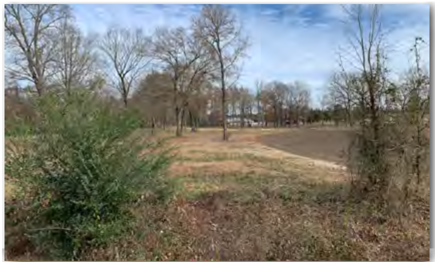
View of site work to increase elevation
