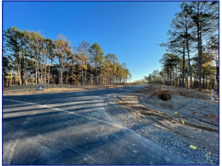
View from intersection of Orchard Ln and Orchard Heights Dr looking E
