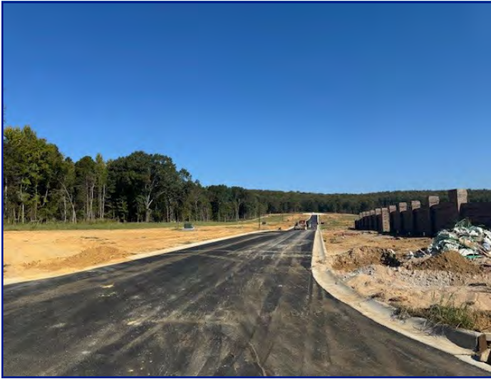
View of subject property looking N
