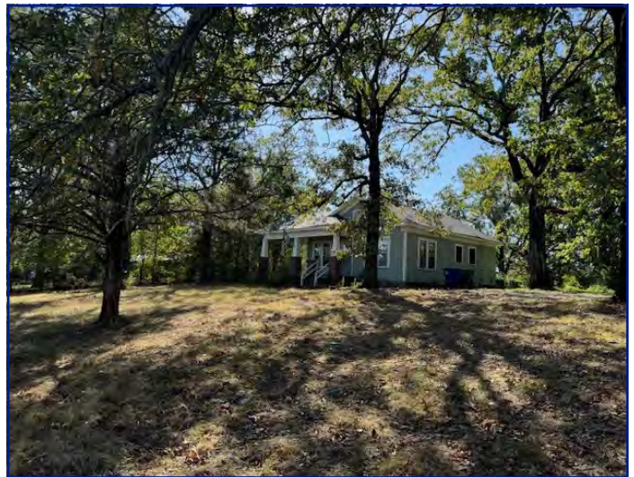
View of subject property facing SE from Meadowlake Rd
