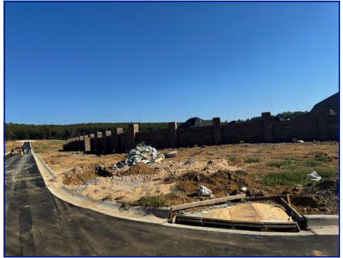
View of subject property looking NE
