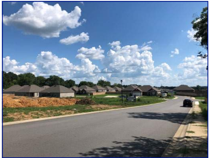
View from subject property looking S along Matthews Meadows Ln
