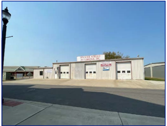
View of subject property from Smith St looking N
