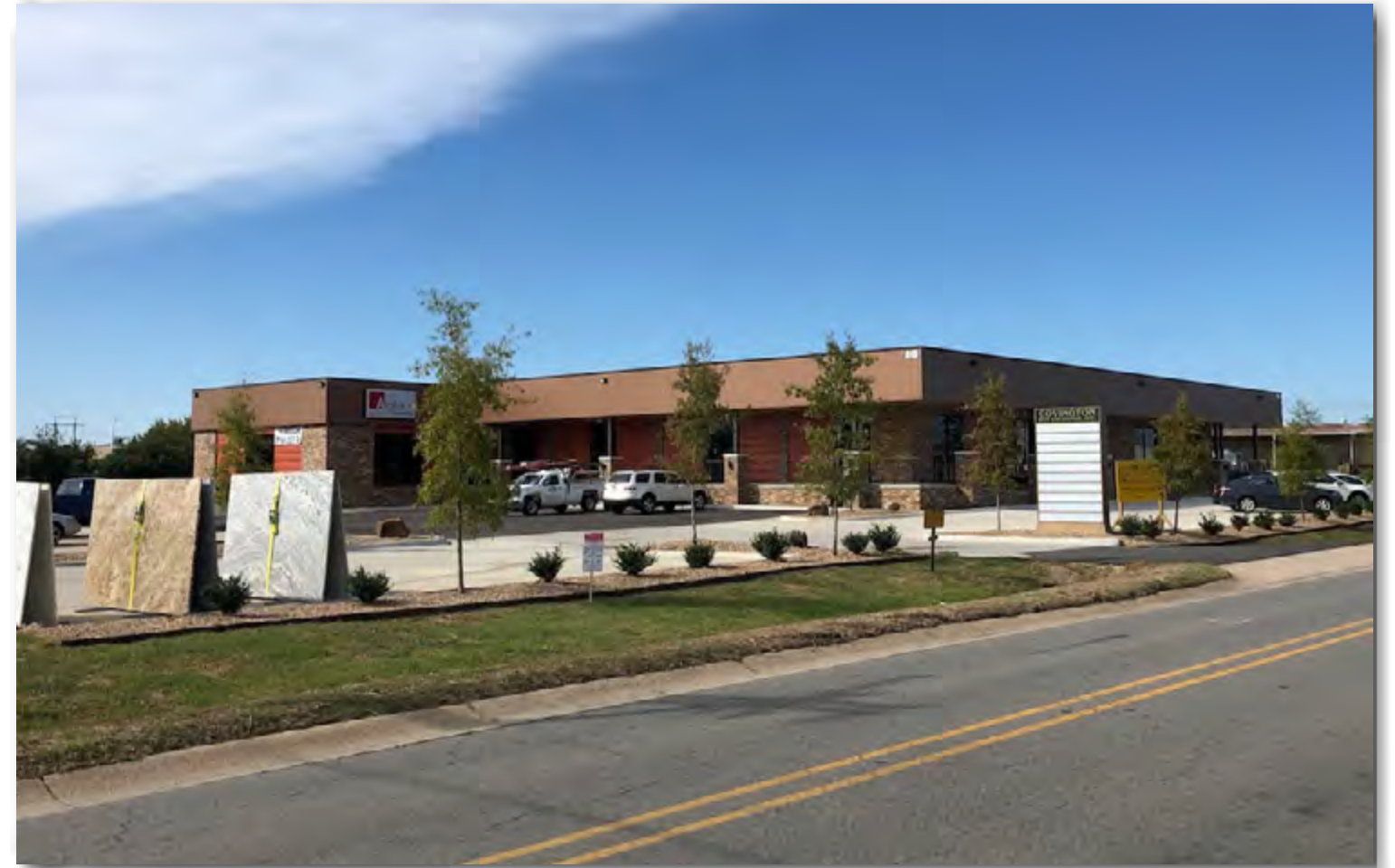
View of subject property from Exchange Ave looking northwest
