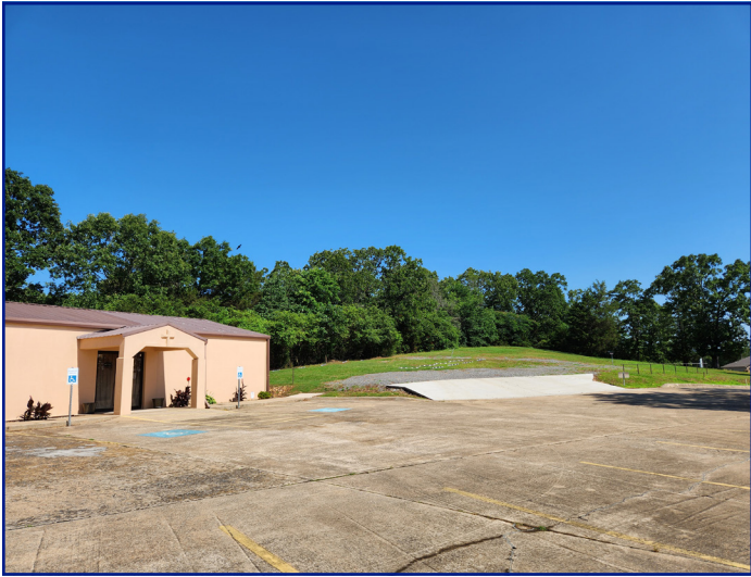
View of subject property from S German Ln looking NW
