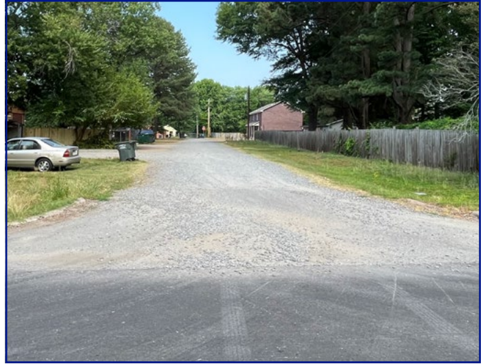
Torreyson St intersection at S Ash St, looking W
