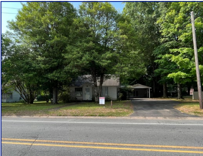
View of front of 1709 Robins St looking S
