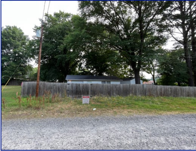
View of rear of 1709 Robins St looking N
