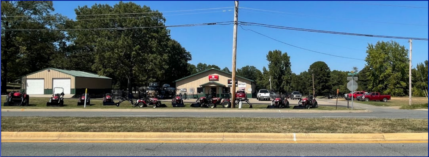
View of subject property from Dave Ward Dr looking N
