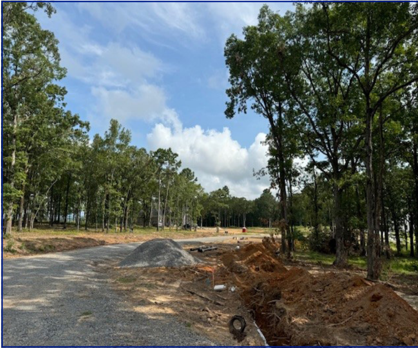
View of road looking N
