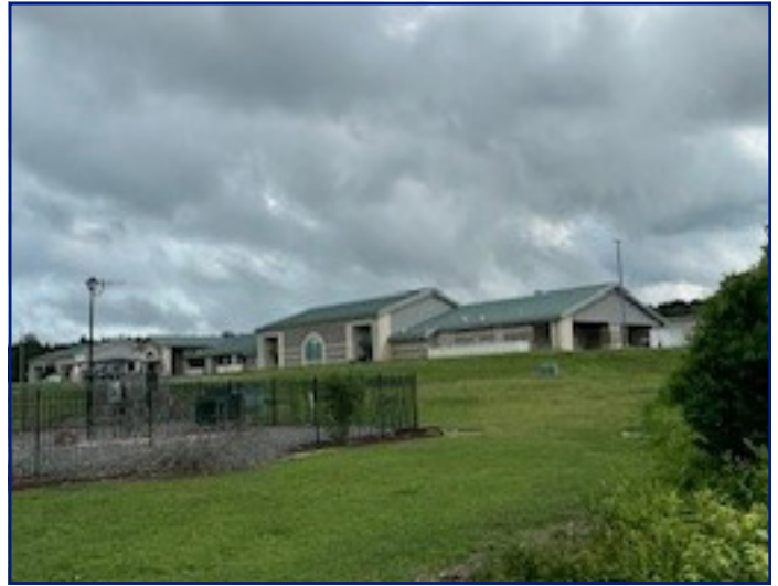
Property adjacent to the N
