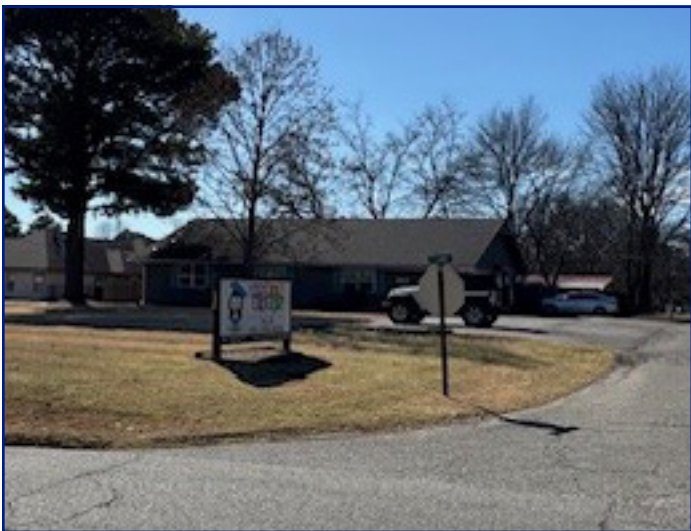
View of subject property looking SW
