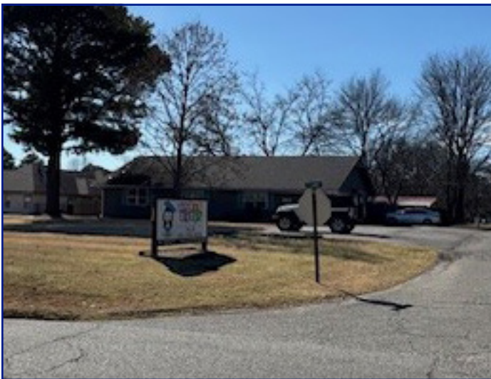
View of subject property looking SW
