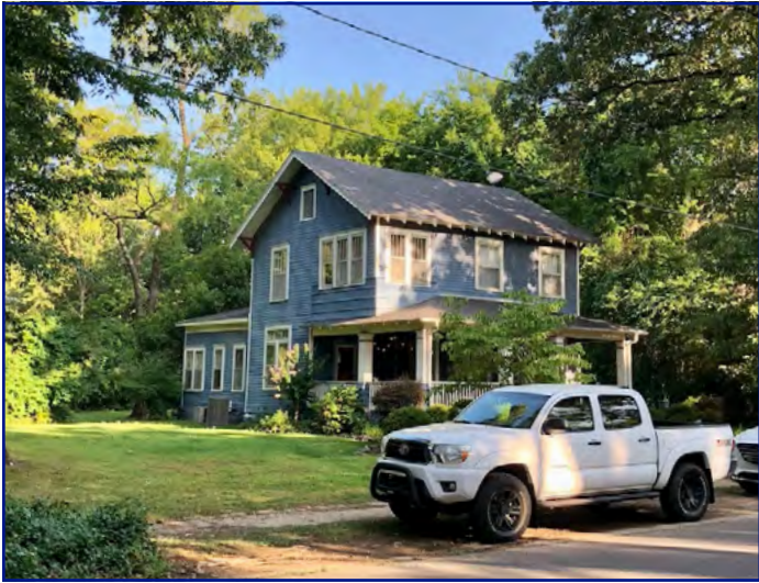
View of property looking NW
