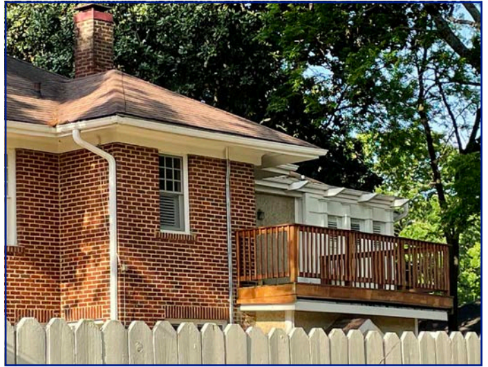
View of rear of subject property from Mitchell St looking SW
