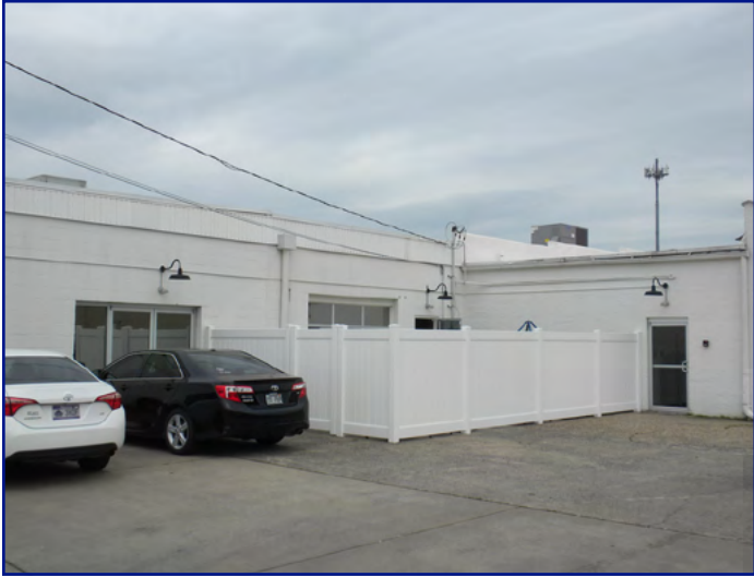
View of fence from parking area looking NW
