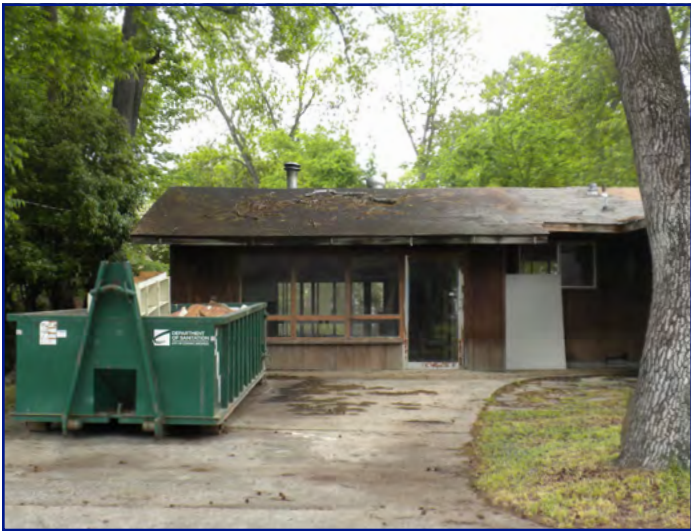
View of subject property looking N
