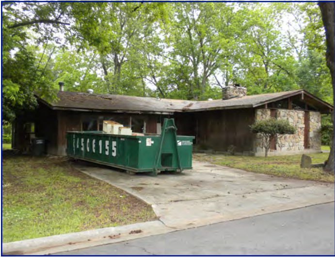
View of subject property looking NE
