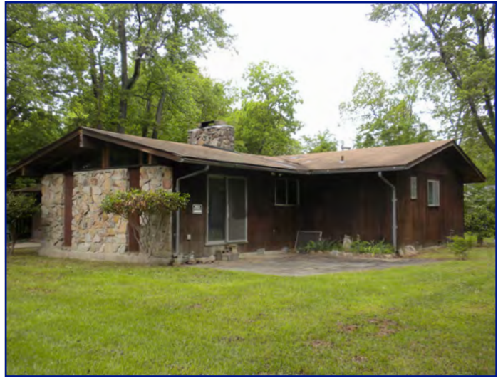
View of subject property looking NW
