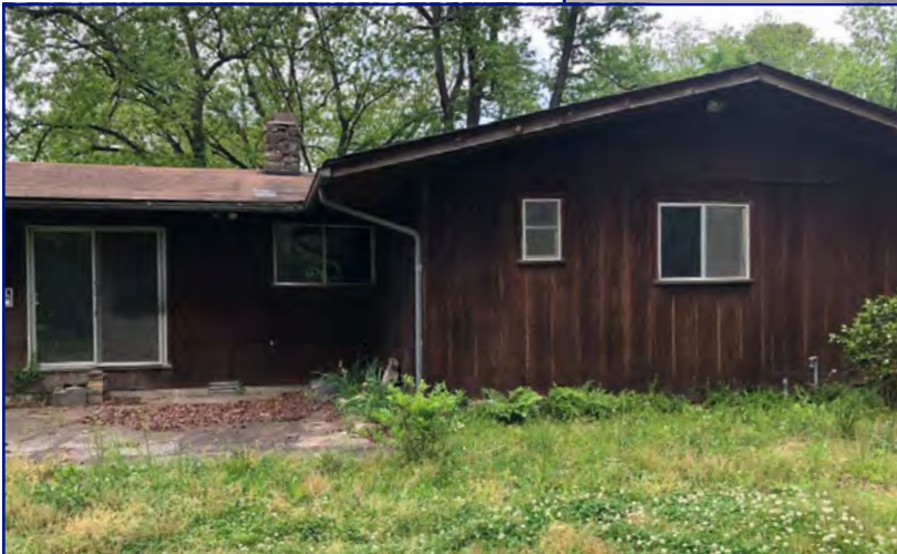
View of east side of house
