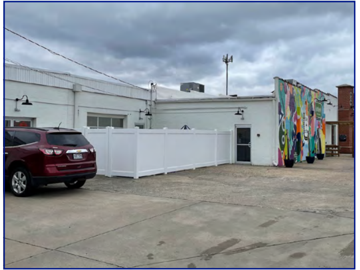
View of fence from parking area looking NW
