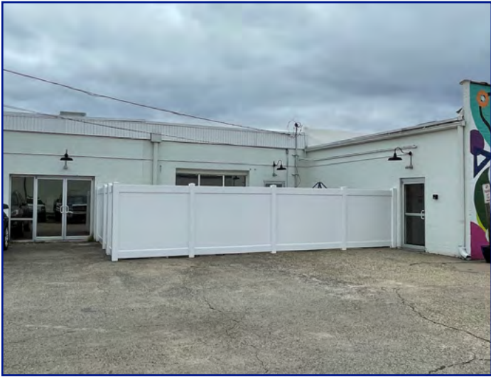
View of fence from parking area looking W
