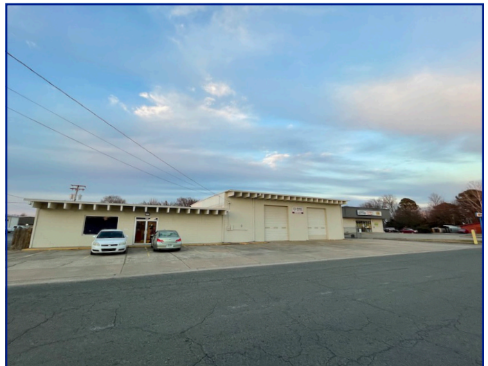
Property adjacent to the N
