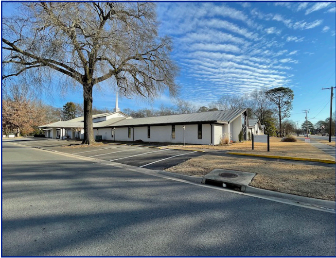
View of subject property from Mitchell St looking NE
