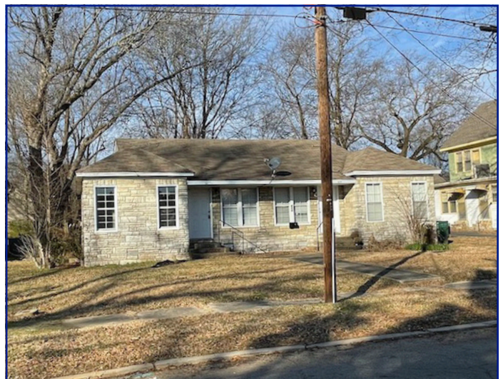
Property adjacent to the N
