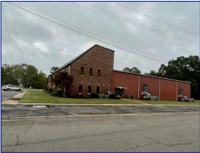
View of existing building from Center St looking E
