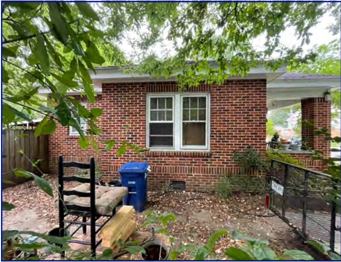
View of W facade of subject property
