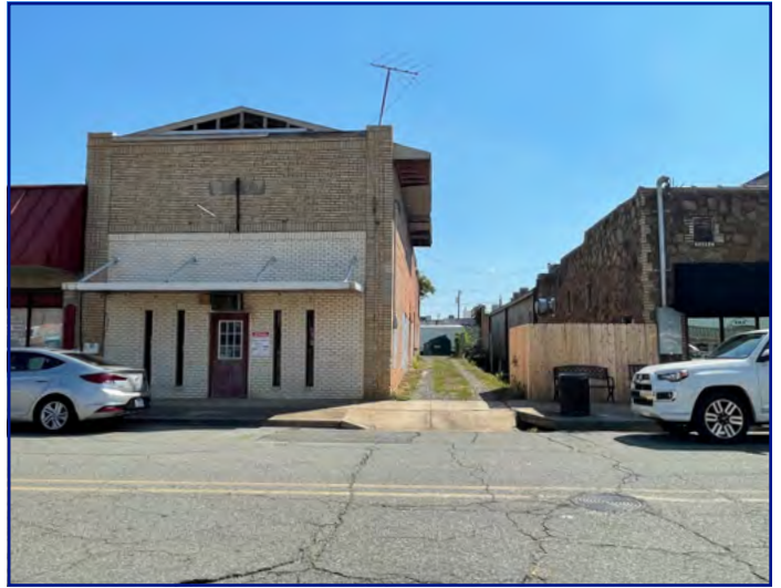
View of subject property from Chestnut St looking E
