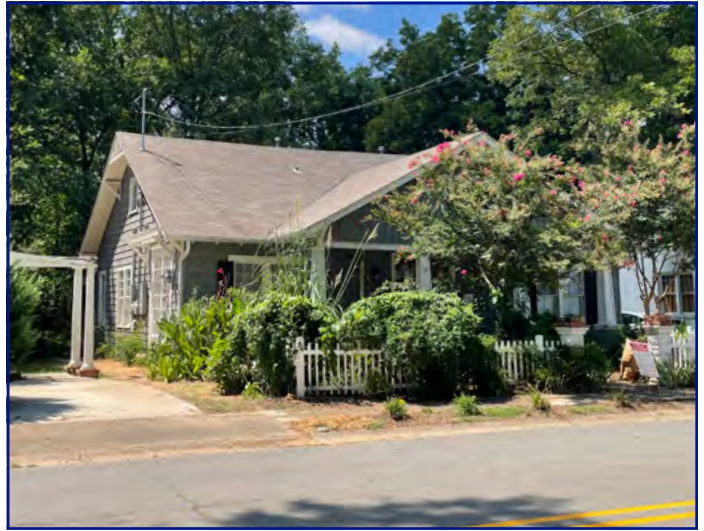
View of subject property from Center St looking NW
