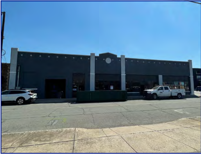
View of subject property from Chestnut St looking E
