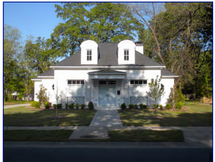
Property adjacent to the N
