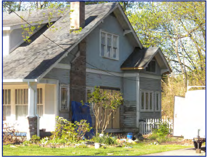
View of subject property looking SW
