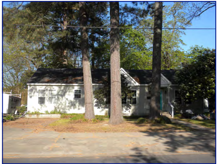
Property adjacent to the N
