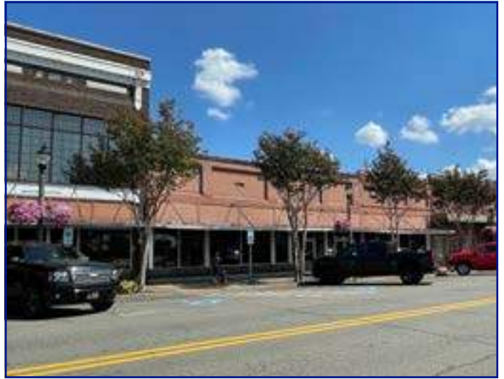
View of subject property from Front St looking SE
