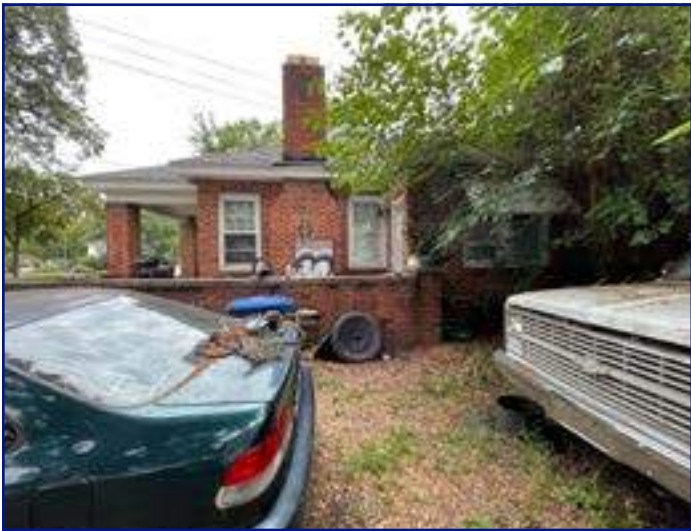
View of E facade of subject property
