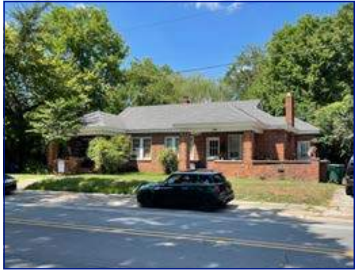
View of subject property from Caldwell St looking NW
