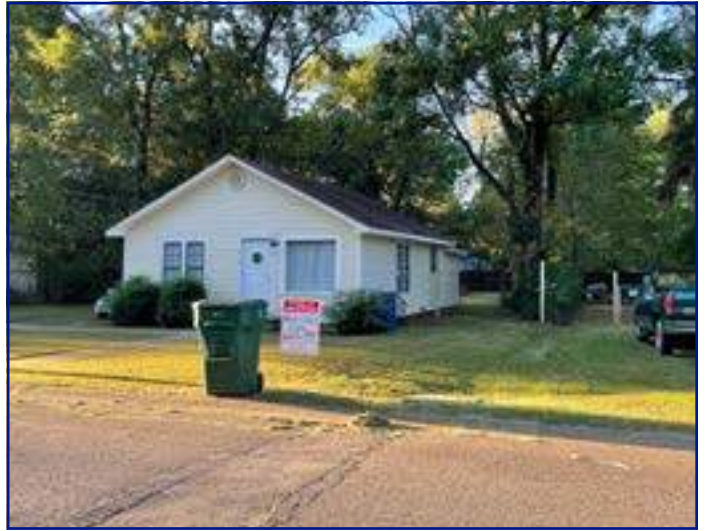
View of subject property from Second St looking SE
