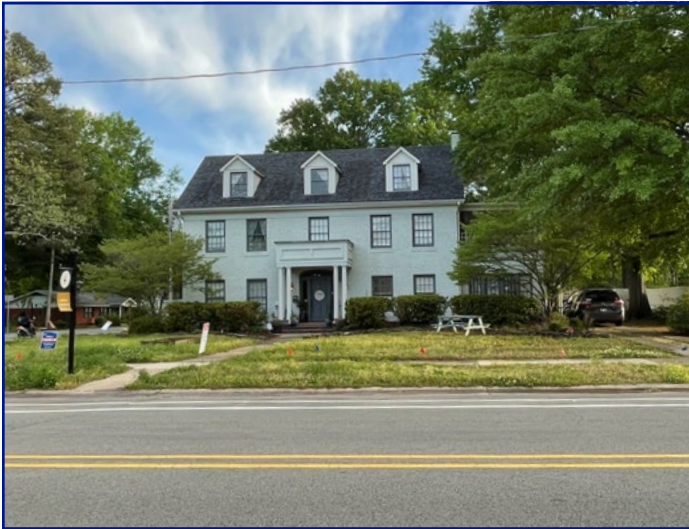
View of 1724 Robinson Ave looking N
