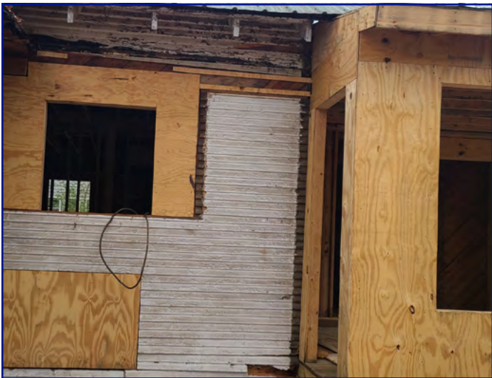
View of addition/work to east side of structure
