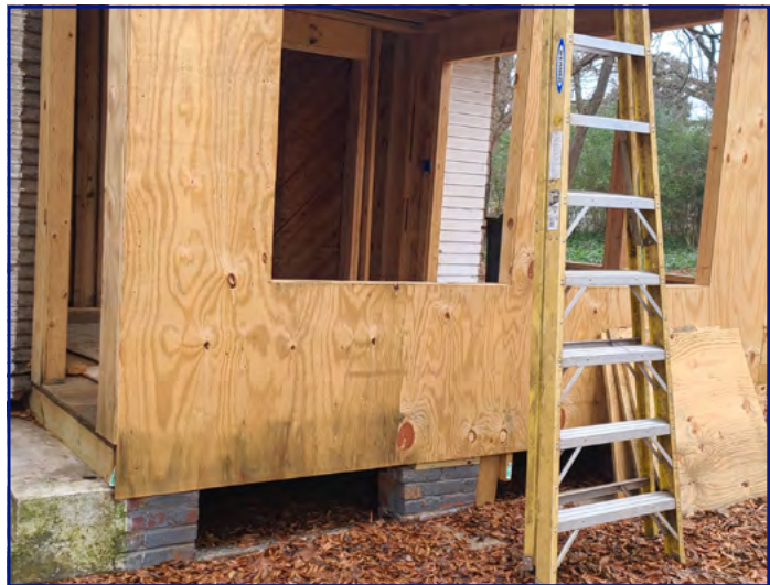
View of addition to east side of structure
