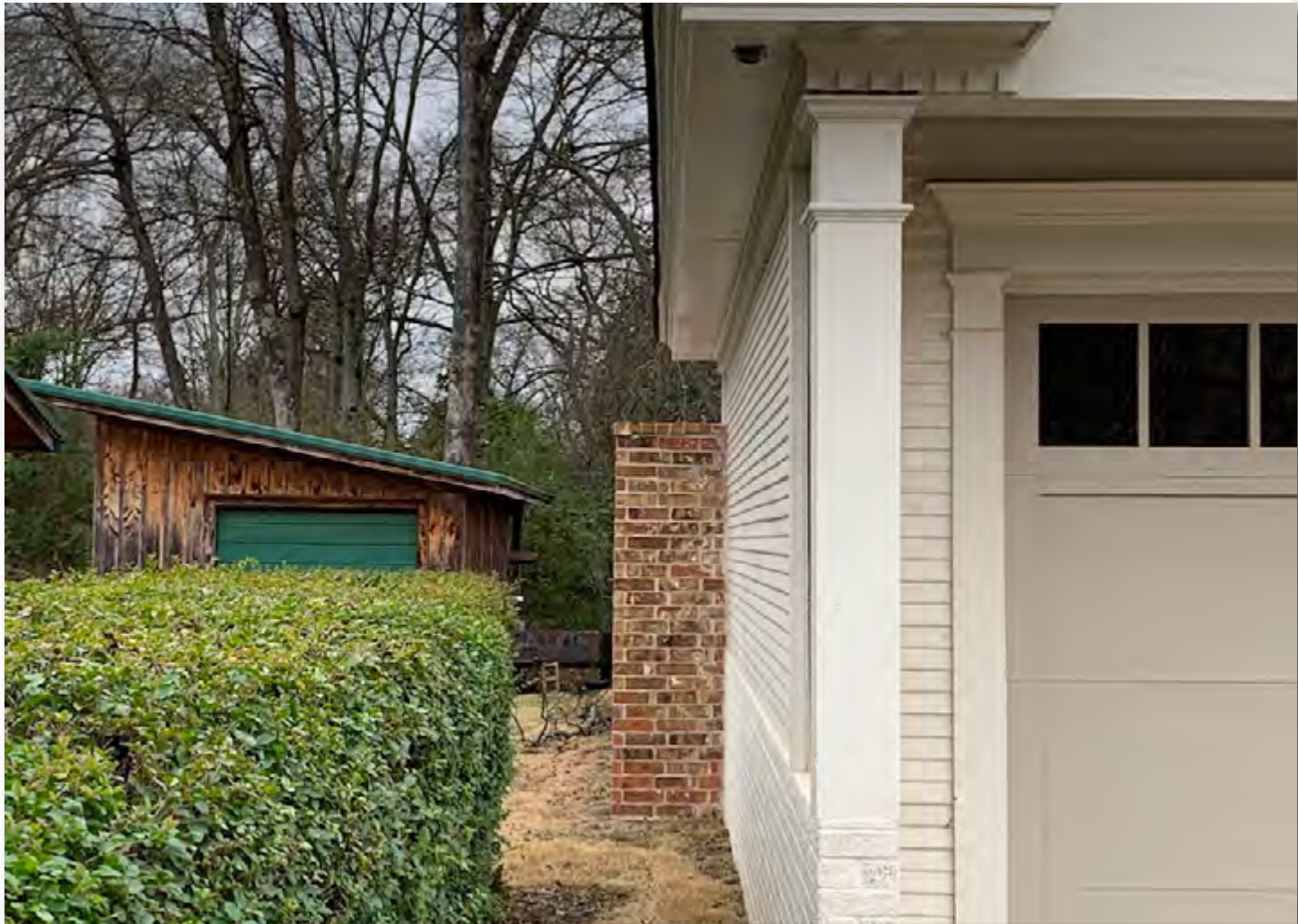
View of wall along south property boundary
