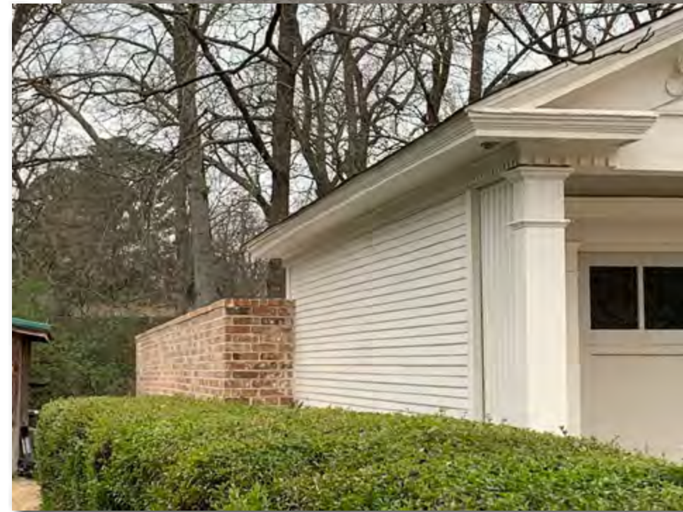
View of wall along south property boundary
