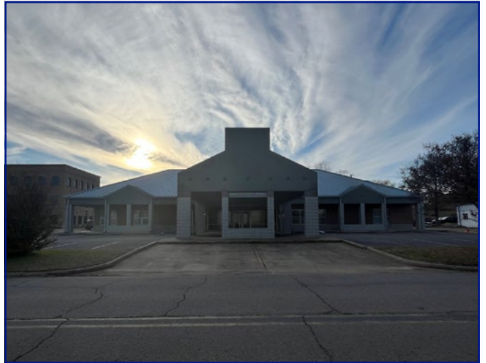
View of subject property from Parkway St looking W
