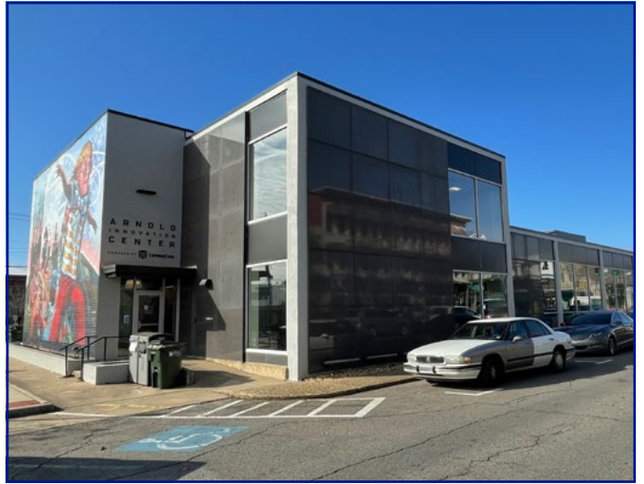
View of subject property from Front St looking NW
