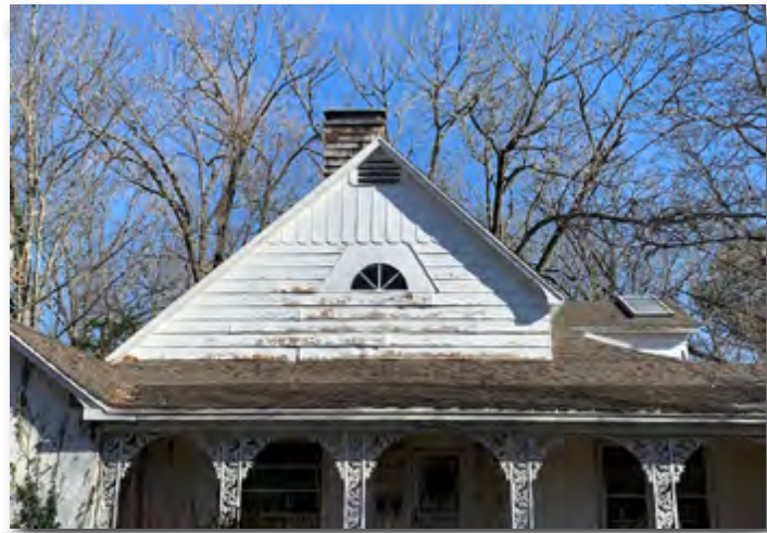
View of roof of subject property
