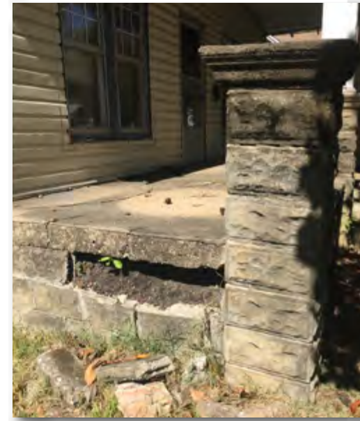
Existing porch, to be replaced
