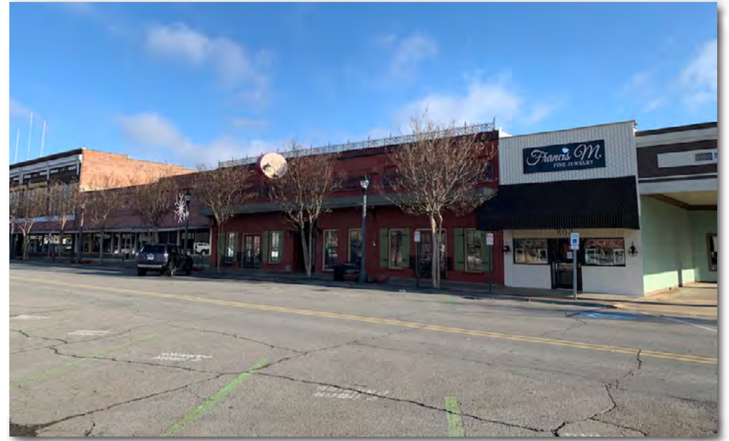
Properties adjacent to the north, along Front St
