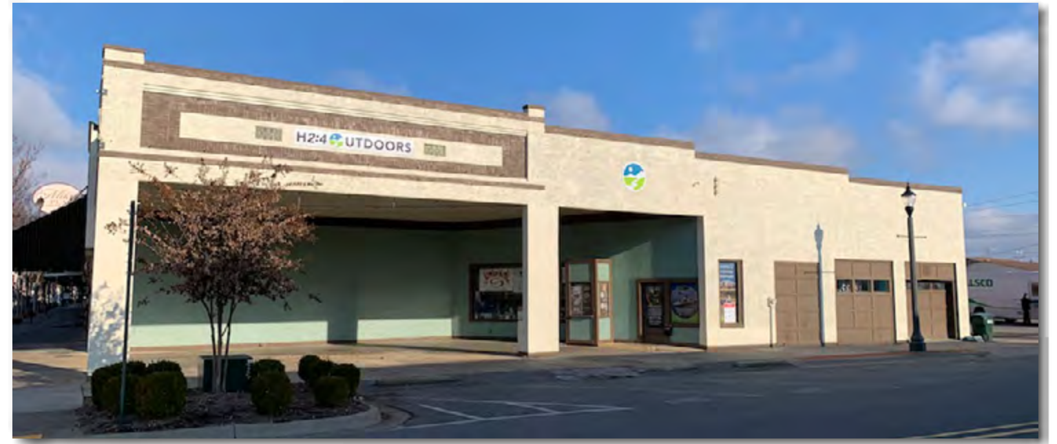
Existing south façade
