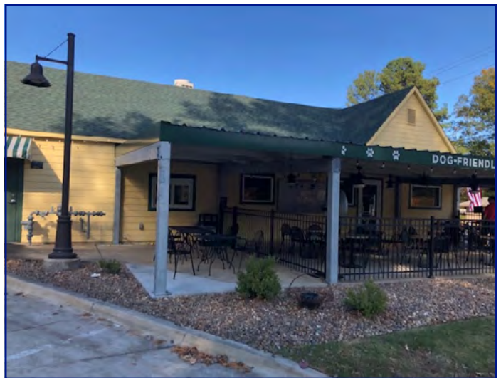
View of subject property from Robinson Ave looking NW
