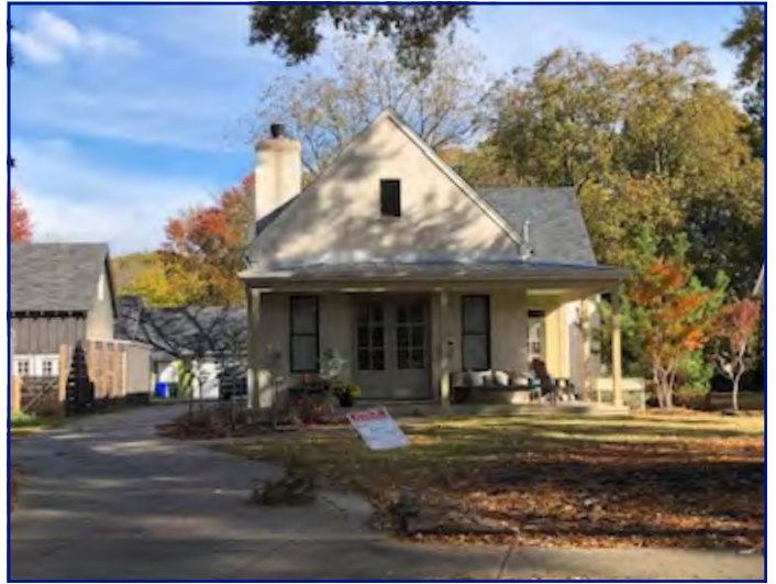
View of subject property from Conway Blvd looking S
