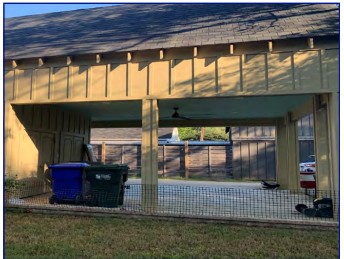
View of carport
