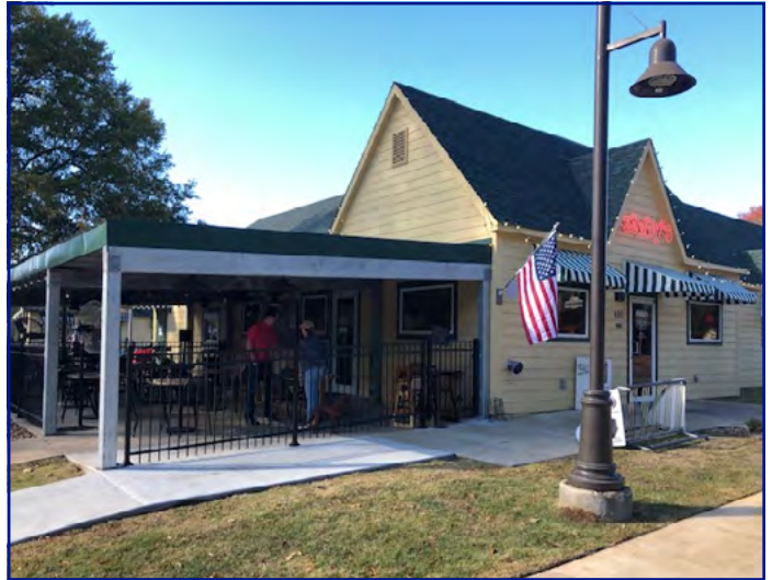
View of subject property from Donaghey Ave looking NW
