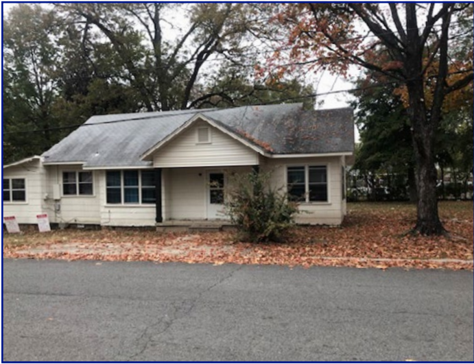
View of subject property from Weems St looking N
