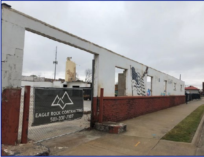
View of subject property from Front St looking NW
