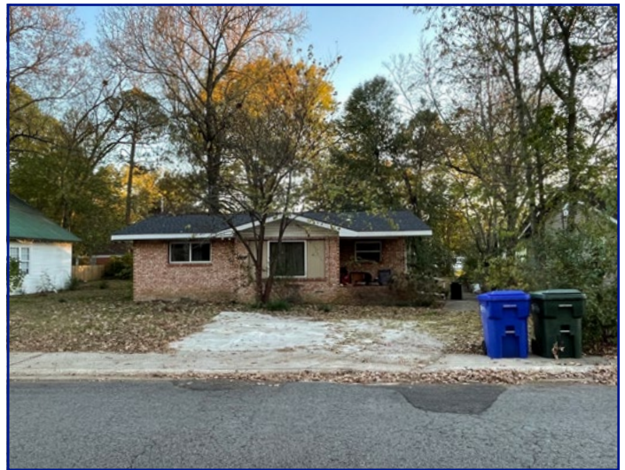
Property adjacent to the S, across Weems St
