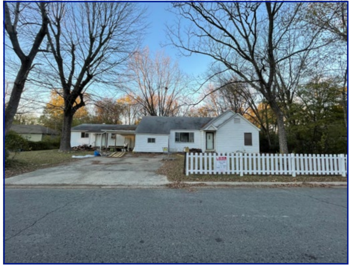
View of subject property from Weems St looking N
