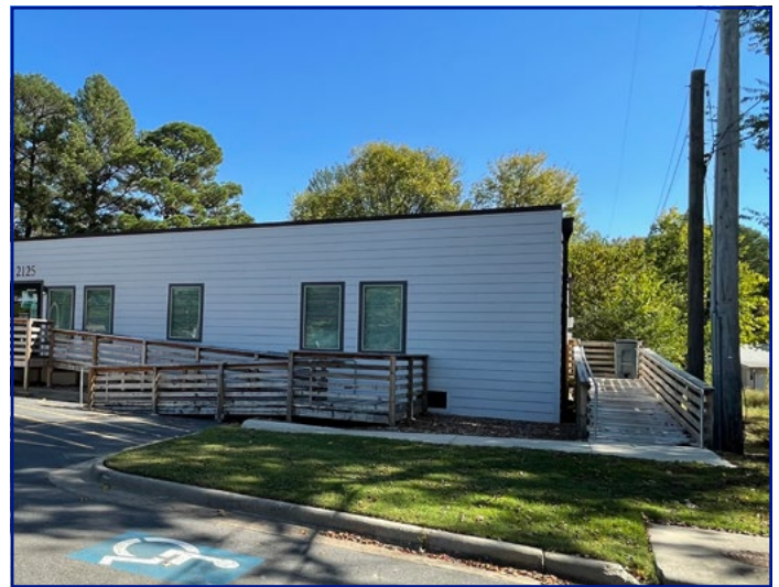
View of south entry to subject property
