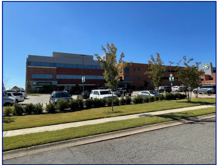
CRMC Medical Office Building SW of subject property
