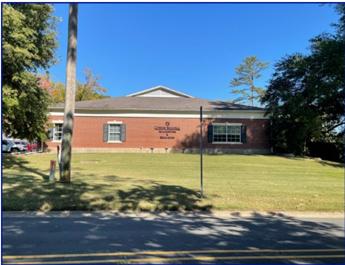
CRMC facility across Robinson Ave to the N
