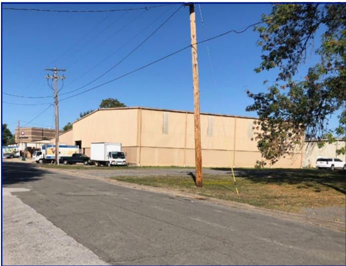
Property to the NW on the north side of 1 st St
