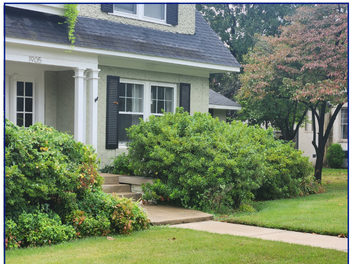
View of porch addition area
