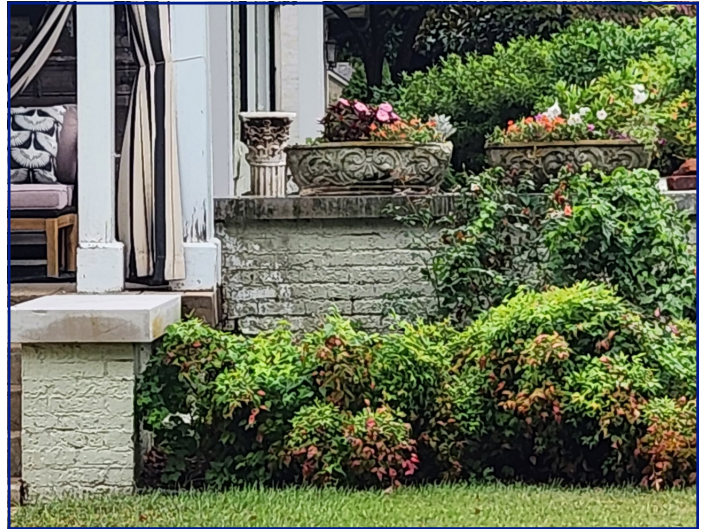
View of porch repair area
