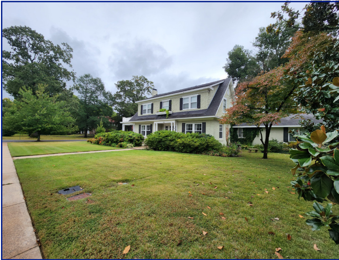
View of subject property facing SE
