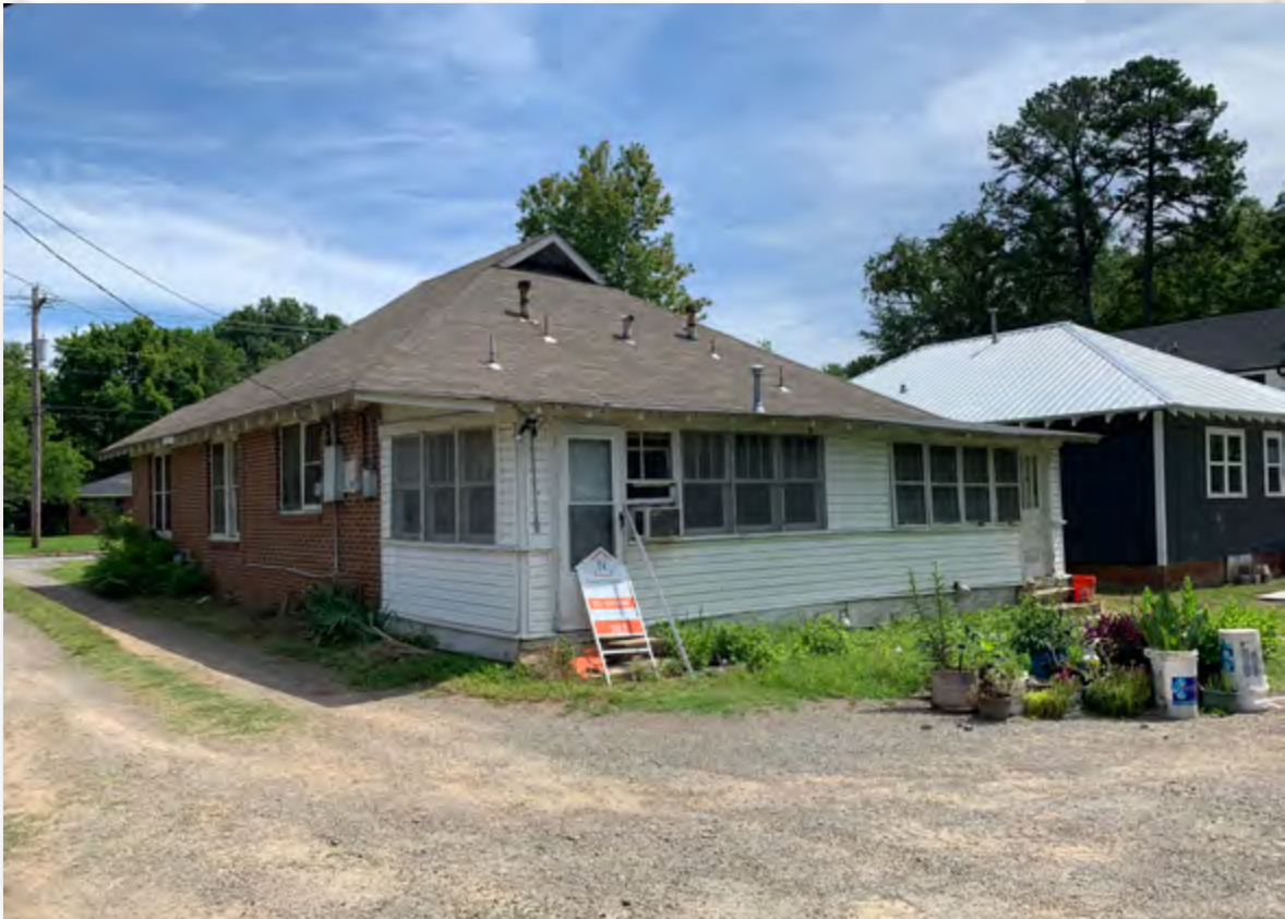
View of existing addition to be removed
