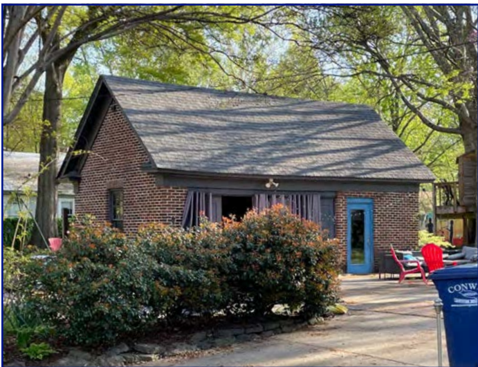
View of accessory structure at rear of subject property
