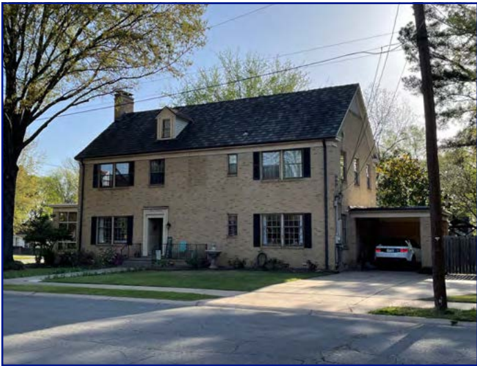
Property adjacent to the N
