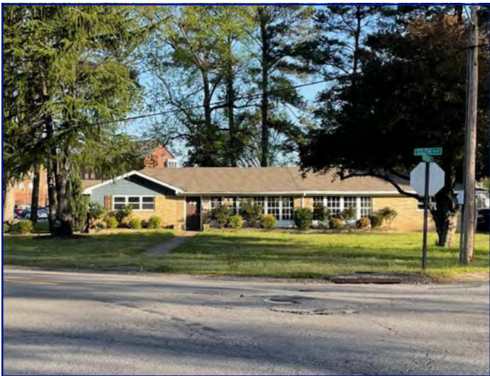
Property adjacent to the NW
