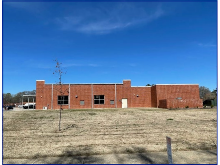
View of subject property from Robins St looking N
