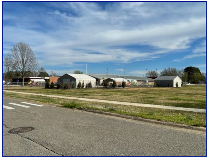
View of subject property from South Blvd looking SE
