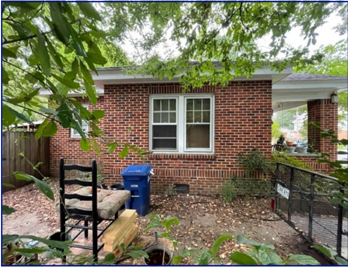
View of W façade of subject property
