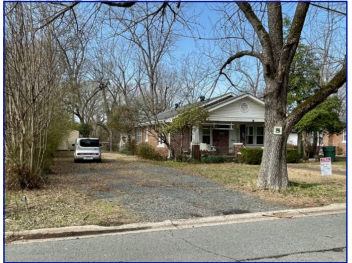
View of subject property from Watkins St looking NW
