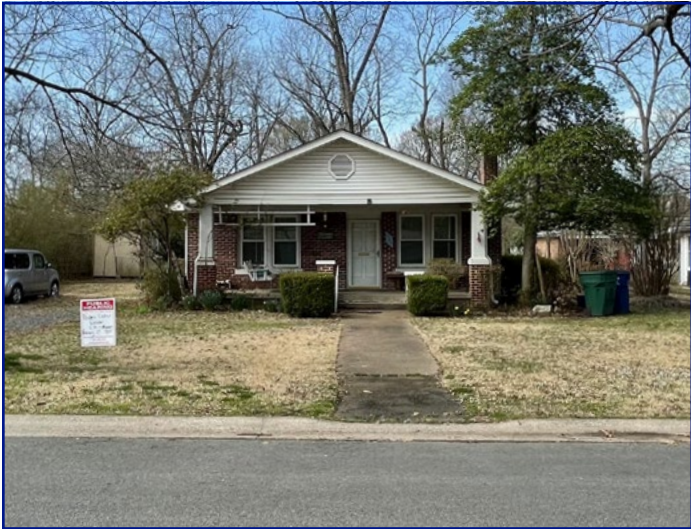
View of subject property from Watkins St looking W
