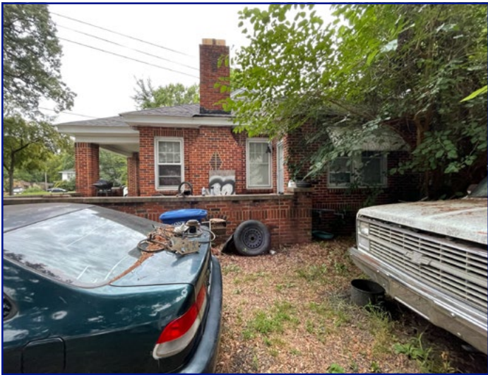
View of E façade of subject property
