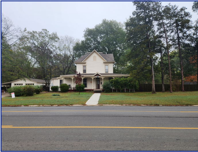
View of subject property facing E
