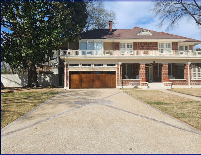
View of subject project property facing N
